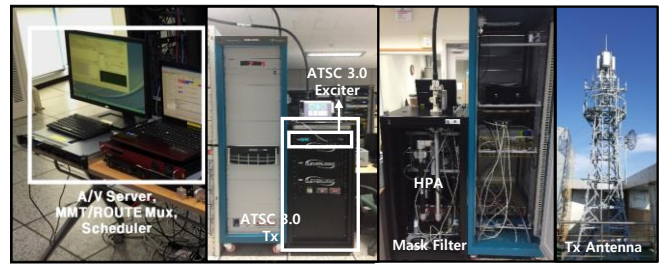
Fig. 18. Facility configurations: Studio/transmitter-side infrastructure [9].
